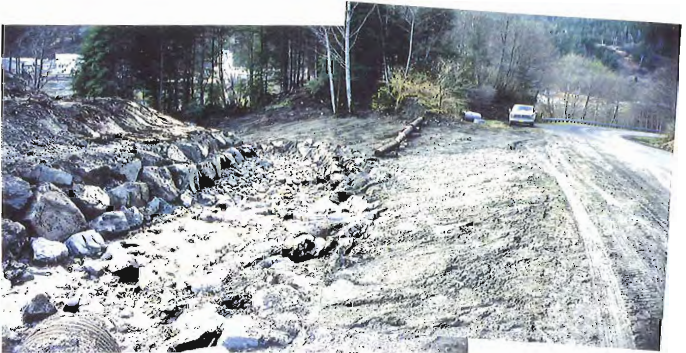
Photo #14: 11/11/99 view looking down the APC/Sitka landfill's surface water drainage ditch just beyond the Sawmill Creek Road's culvert discharge, showing the gentle roadside embankment and barrier logs placed well away from the road (refer to Photo #15).
