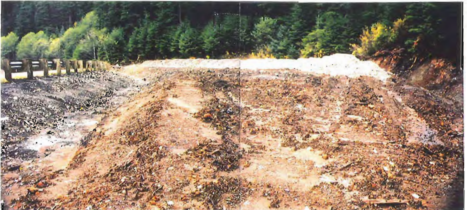
Photo #26: 10/20/99 view looking north across the APC/Sitka landfill's northeastern area, showing the surface water ditchlines along both sides of the fill and the stockpiled loads of crushed-concrete fill (about 200 c.y.) waiting to be spread across the top surface and then covered with 4" of final surface soil.
