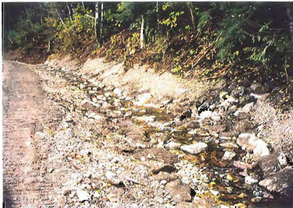
Photo #20: 10/20/99 view of the main creek coming into the drainage ditchline along the upland side of Sawmill Creek Road, showing the large rock placed along its entrance to protect against erosion.
