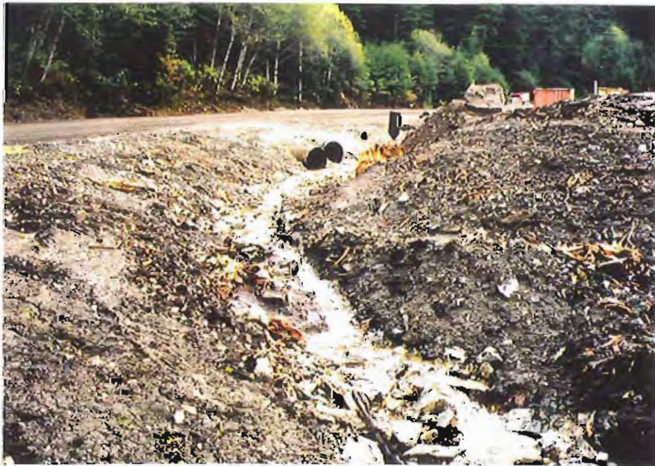
Photo #22: 10/20/99 view looking upstream around the APC/Sitka landfill's northwestern corner, showing the conditions prior to any preparation work for placement of its 30-mil membrane liner. The arrow points to a large stump that was removed the next day, to move the drainage centerline further away from the road.
