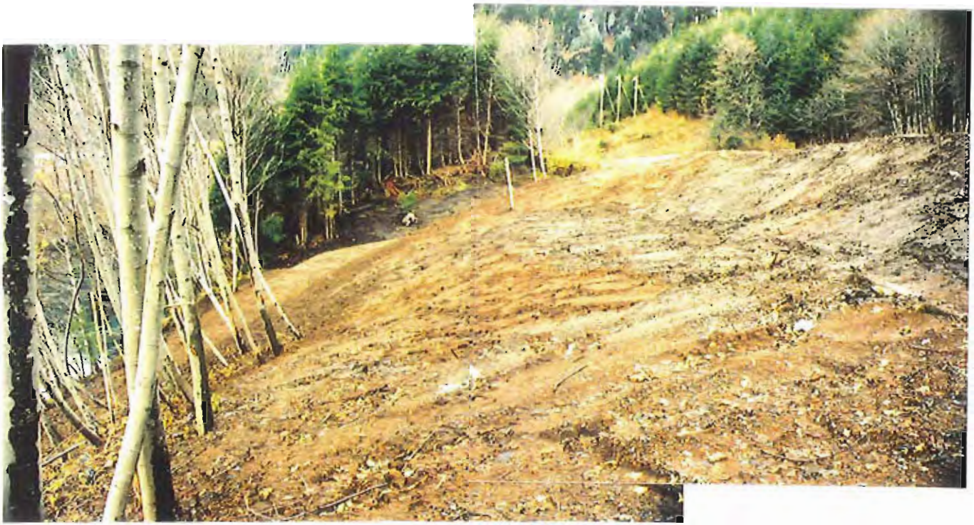
Photo #69: Closer view of the APC/Sitka landfill's northwestern embankment area on 11/11/99, showing the completed 6"-thick soil cover across the lower access path to the leachate sampling site (see next 5 photos).
