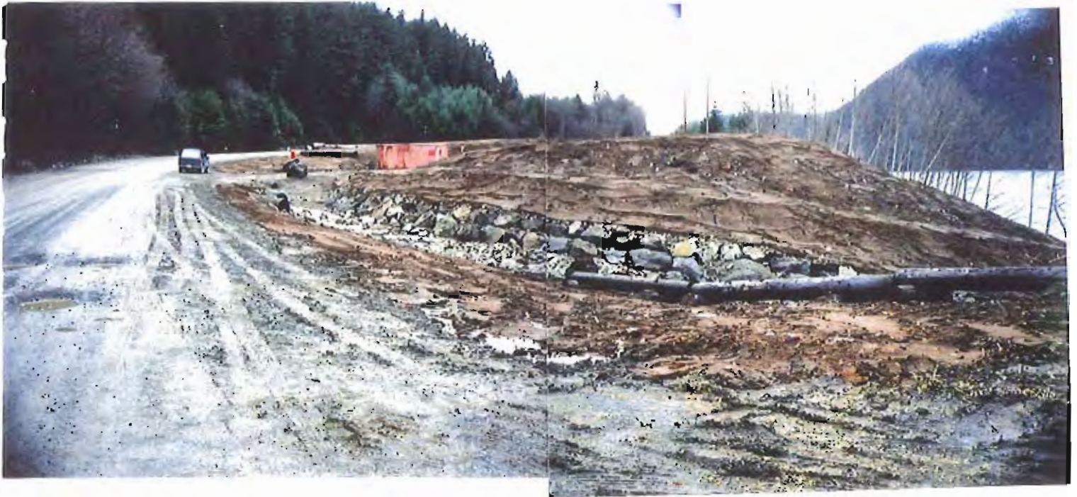
Photo #13: Looking across the northwestern end of the APC/Sitka landfill, showing the gentle banks of the surface water drainage ditchlines along Sawmill Creek road (see next photo).
