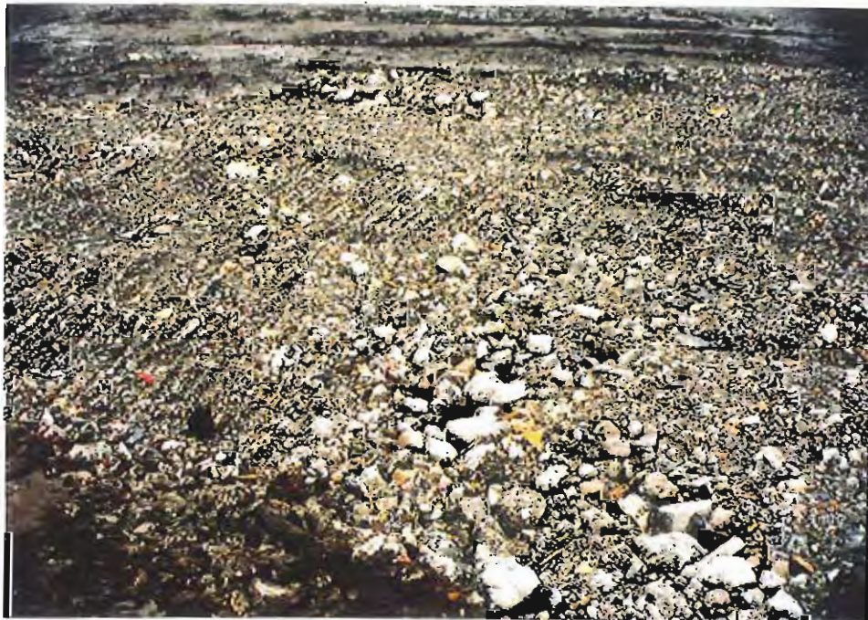
Photo #24: Closer view of the top surface of the 1.5'-thick lift of crushed concrete fill being added to the top of the APC/Sitka landfill surface, showing its clean and porous appearance (10/20/99).
