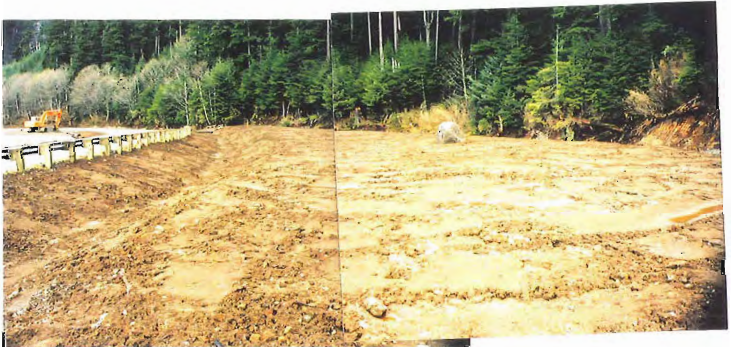
Photo #6: Looking across the middle portion of the APC/Sitka landfill's northeastern disposal area on 11/23/99, showing the newly created drainage ditch along Sawmill Creek Road.
