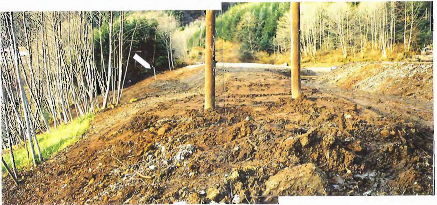
Photo #68: Looking across the APC/Sitka landfill's northwestern end, showing the final 6"-thick soil cover already in place across its outer embankment (arrow points to the former asbestos fence corner post that has been left in place for reference). Its upper surface still needs a 18" lift of crushed concrete and a final 6"-thick cover of soil before it is completed.
