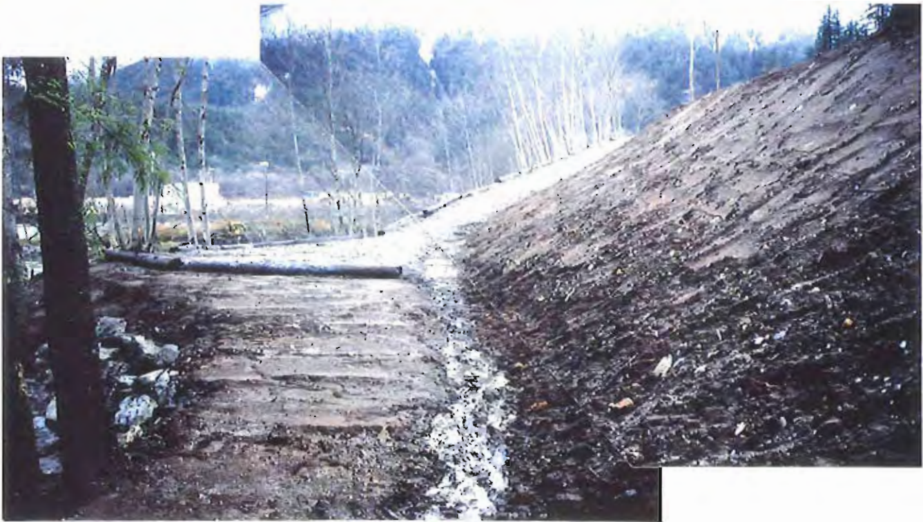
Photo #87: 11/23/99 view of the APC/Sitka landfill's embankment toe near its southern end, showing the drainage ditch for the surface water coming from the embankments and roadway.
