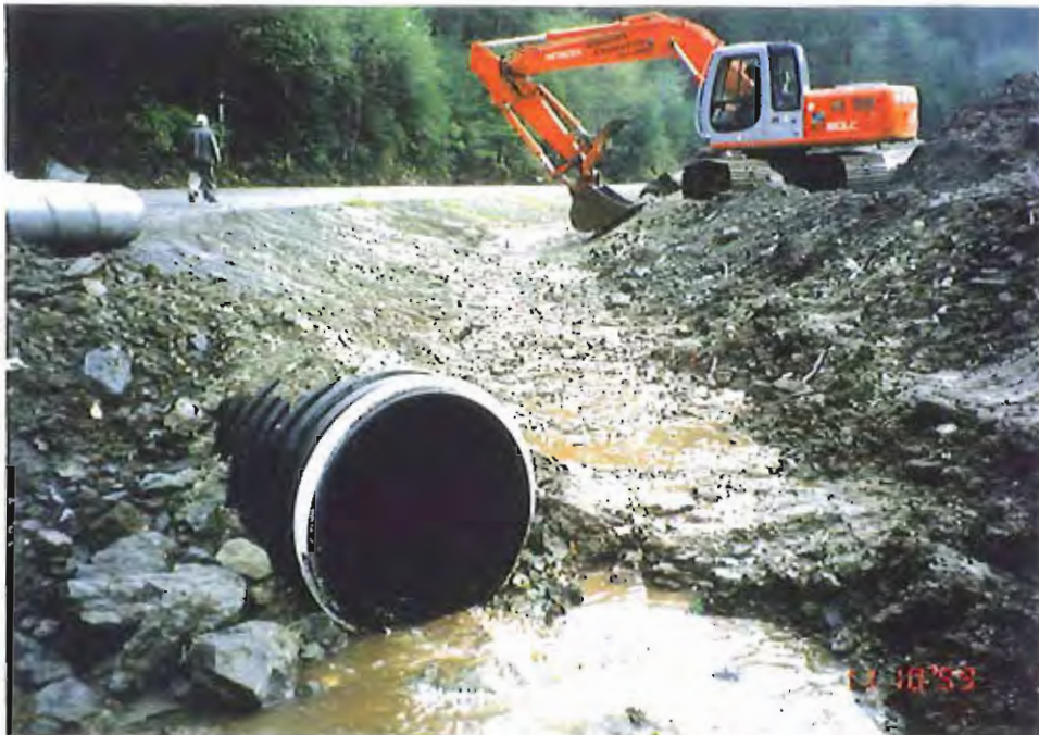
Photo #3: 10/11/99 view of the new 3'-dia. culvert discharge from across the Sawmill Creek Road, looking up the roadside drainage ditch being prepared for placement of the 30-mil membrane (see next photo).
