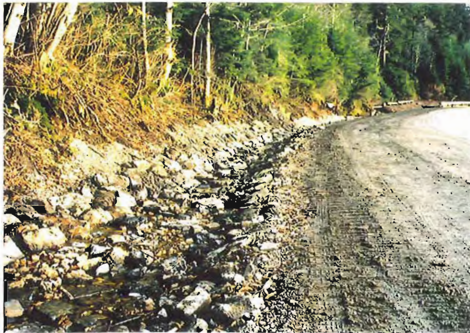
Photo #60: Closer 11/11/99 view of the upslope surface water drainage ditch along the Sawmill Creek road, showing the completed placement of armor rock along the sides of the ditch (compare with Photo #20, page A11).
