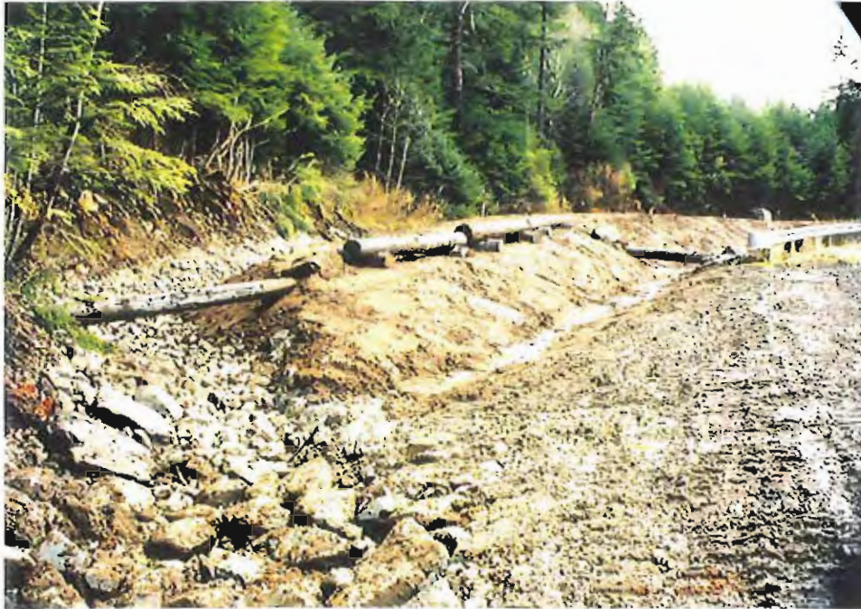
Photo #61: 11/11/99 view looking southeast across the lower end of the APC/Sitka landfill's northeastern disposal area, showing the completed ditchlines, final soil cover and roadside log barriers.
