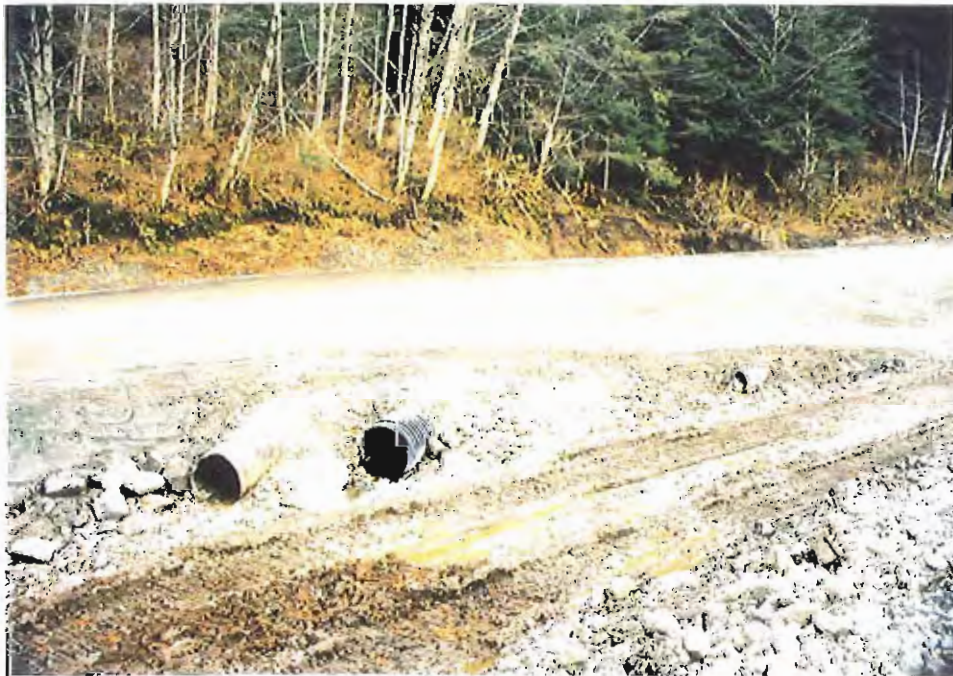
Photo #12: 11/11/99 view of the 3'-dia culvert discharges along the northwestern end of the APC/Sitka landfill. The new culvert is on the right site (see next two photos).
