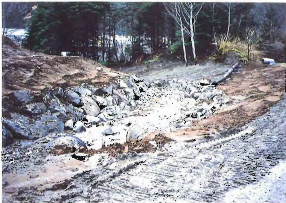
Photo #78: Looking down the open surface water ditch around the APC/Sitka landfill's northwestern end on 11/23/99, showing the roadside culverts and the large rock lining both sides of the ditch (compare with Photo #34 on page A18).
