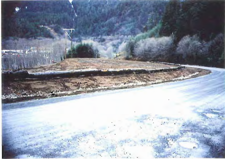
Photo #83: Looking northwest across the upper surface of the APC/Sitka landfill site on 11/23/99, showing its completed soil extending over the sides of the roadside ditchline, and the barrier logs along the top of the ditchline embankment (compare with the photos on page A23).
