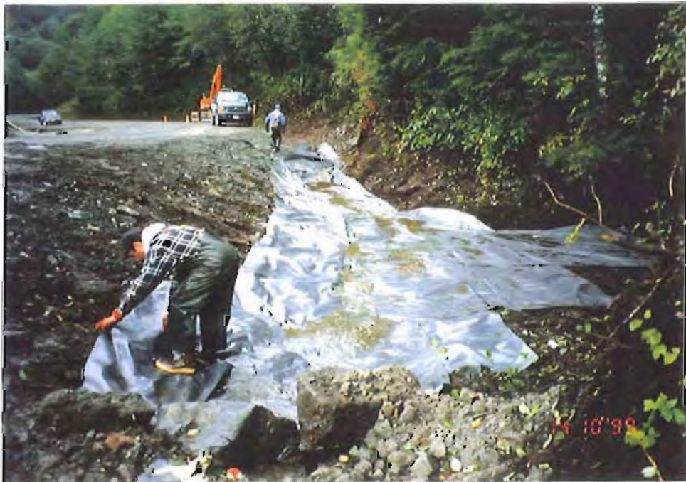
Photo #16: Earlier 10/14/99 view of the 10'-wide by 30-mil membrane liner being placed along the Sawmill Creek Roadway's upslope drainage ditch (compare with Photo #9).
