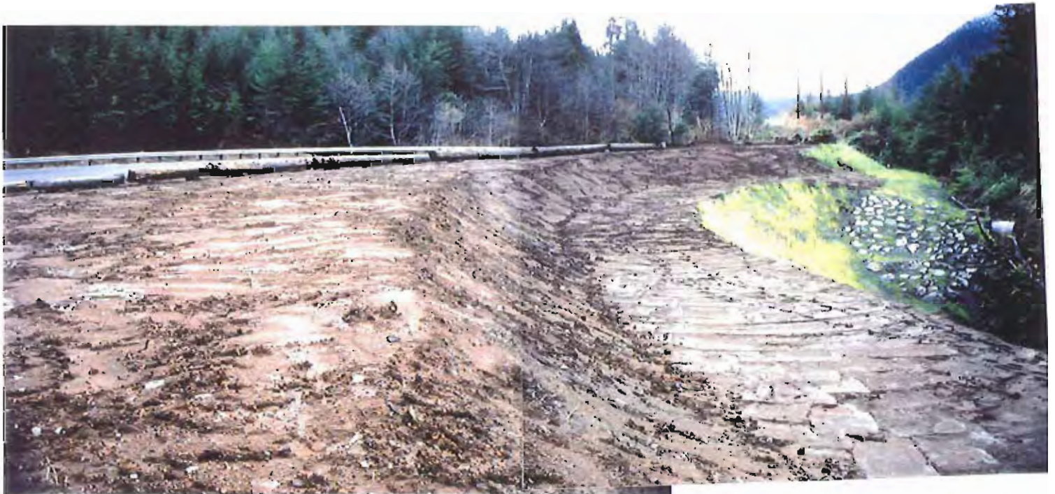
Photo #82: 11/23/99 view of the APC/Sitka landfill's southeastern end, showing its completed final soil cover along the top and upper embankment surfaces, and the barrier logs along the roadside edge of the site (compare with the photos on page A26 & A28).
