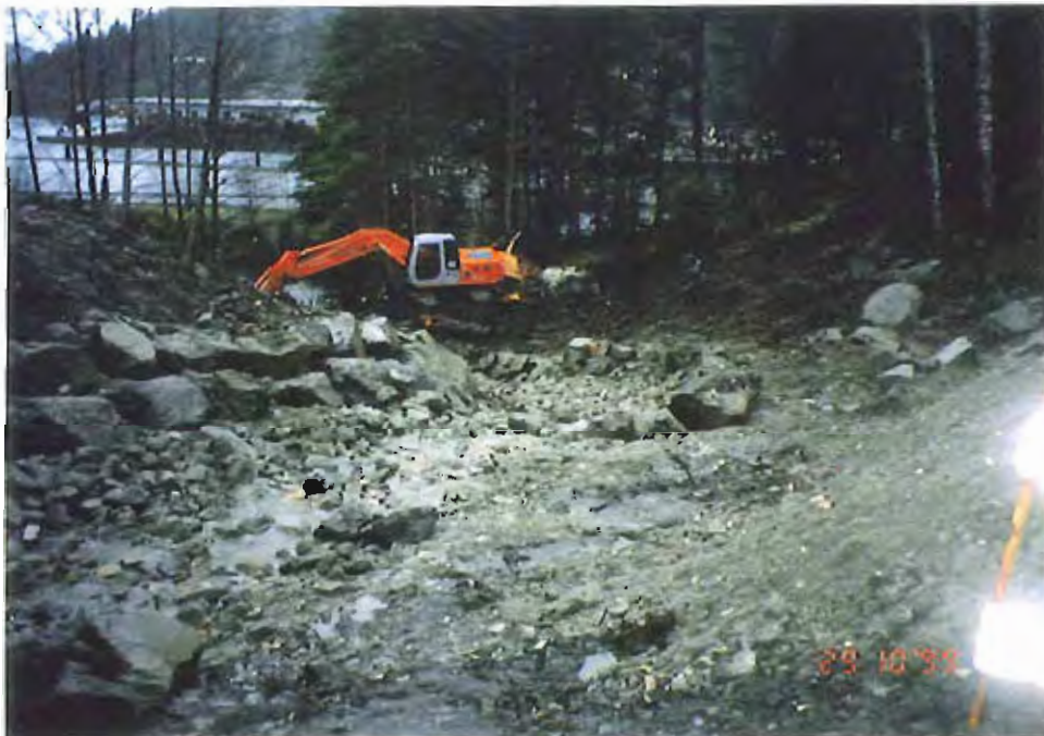
Photo #36: 10/29/99 view looking down the turn in the APC/Sitka landfill's northwestern ditch, showing the 20'-wide by 30-mil membrane liner now completely covered with protective rock (compare with Photo #34, page A18).
