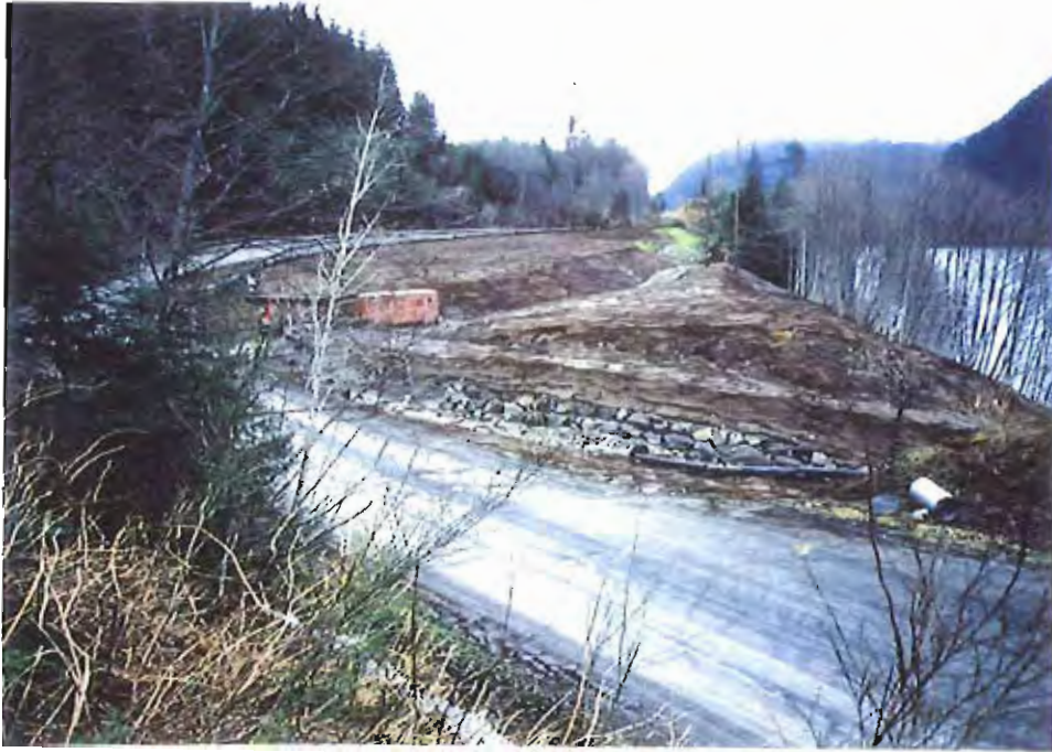
Photo #75: 11/23/99 view looking southeast across the APC/Sitka landfill, showing its entire top area and northwestern embankment to be completely covered with a 6"-thick soil layer.
