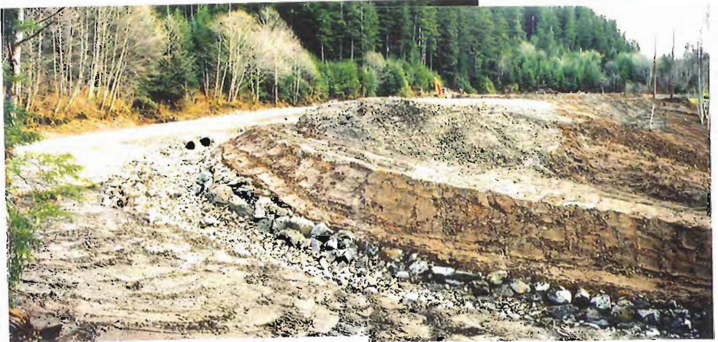
Photo #38: 11/11/99 view of the APC/Sitka landfill's northwestern ditch, now completed.
