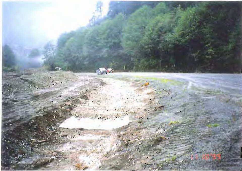
Photo #17: Earlier 10/11/99 view of the 10'-wide by 30-mil liner having been placed in the downslope surface water drainage ditch along Sawmill Creek Road, with a 6"-thick layer of rock over the membrane for protection against erosion (compare with Photo #2).
