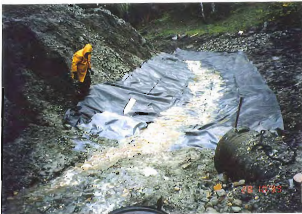
Photo #34: Initial placement of the 20'-wide by 30-mil membrane liner in the APC/Sitka landfill's northwestern ditch on 10/28/99. Arrow points to where the liner section already beneath the culvert discharge has been lapped over the end of the new liner.
