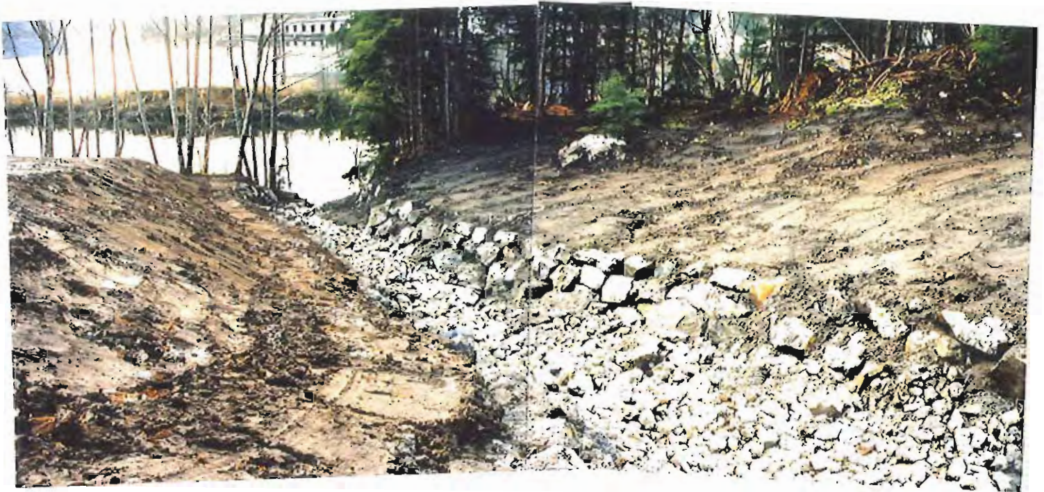
Photo #40: 11/11/99 view looking down the APC/Sitka landfill's northwestern ditchline, showing the completed soil placement and landscaping along both sides of the ditch. Also shown are the large armor rock along the sides of the ditch, and the 6"-8" rock completely covering the ditch bottom for erosion control.
