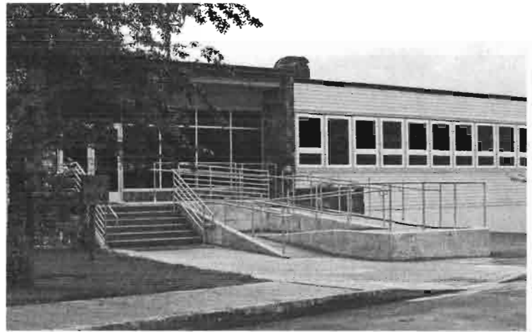
Front Entrance includes ADA accessible ramp
